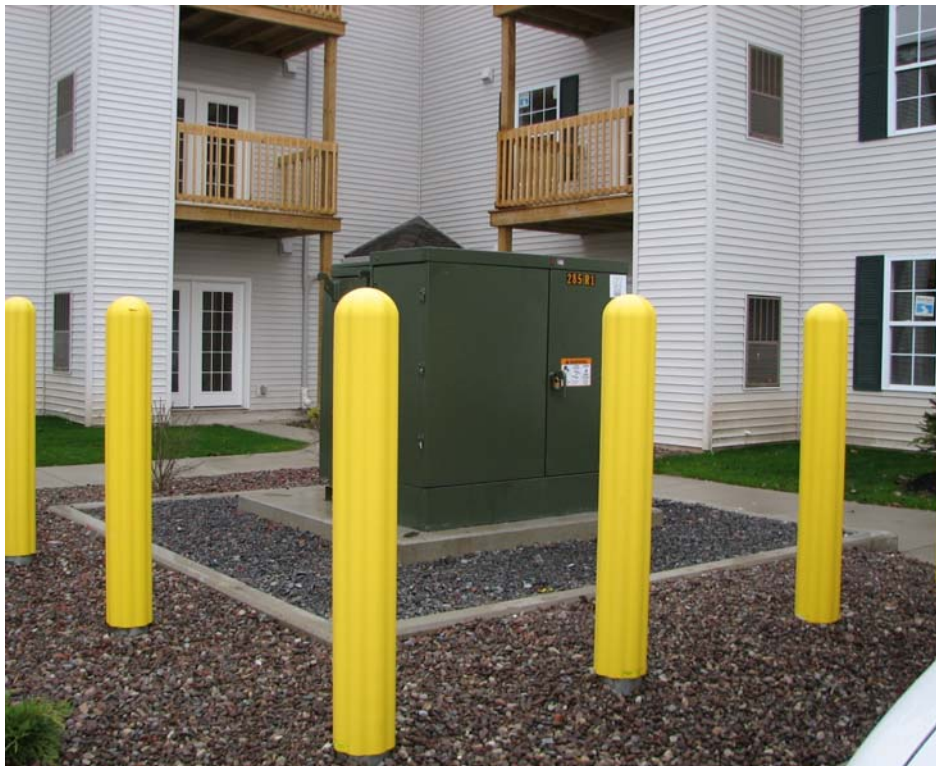
PICTURE OF BOLLARD INSTALLATION for PADMOUNT TRANSFORMER WITH OIL CONTAINMENT FOUNDATION
