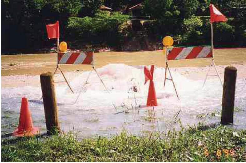
Figure 9-5. Combined sewer overflow near a stream.
