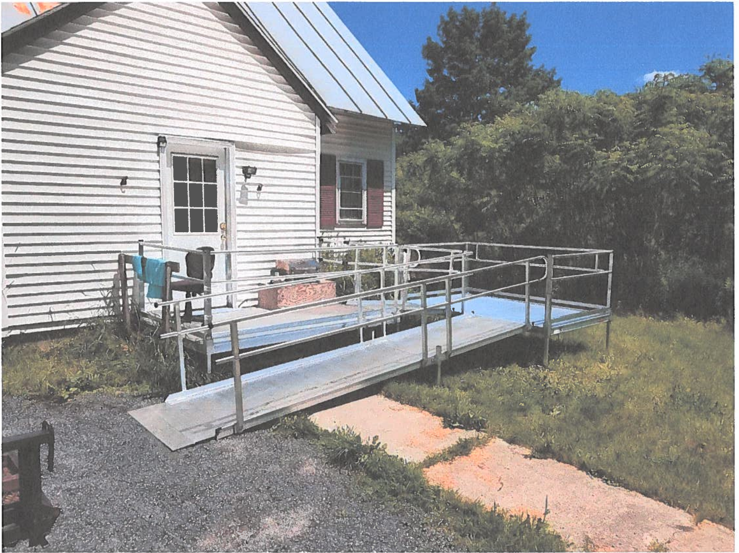
Figure 2. 1336 County Rd. Windsor
