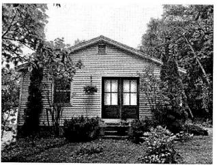
Replace single doors (82 3/4" h x 36"w) at opposite ends of house with double doors (82 3/4" h x 75"w) – replace existing header with longer header (above and below).
