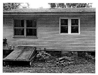
Replace 1 exisiting window (34" h x 34" w) in kitchen with 2 new construction windows (36" h x 58"w) replace existing header with longer header (if required).
