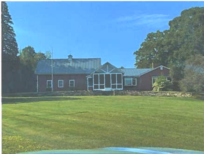
Image 2: BACK ELEVATION VIEW OF GARAGE ROOF
