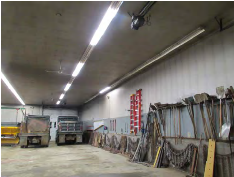
Six circuits control main 4' lighting which allow for optimal control in any situation.
