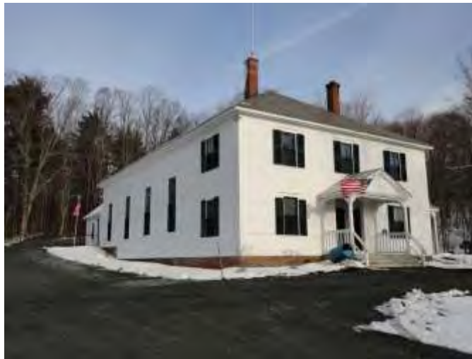
Figure 1. Meriden Town Hall
