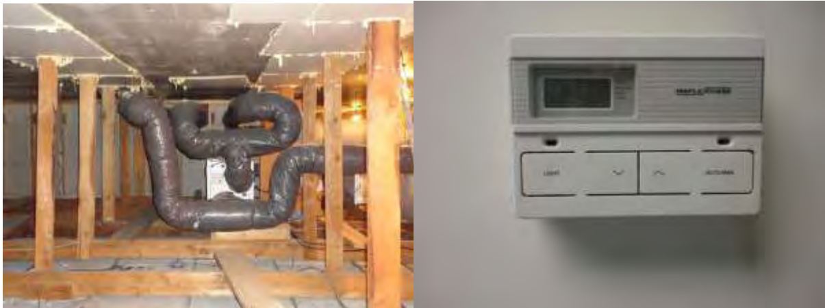
Figure 7. Air-to-air heat exchanger and digital thermostat
