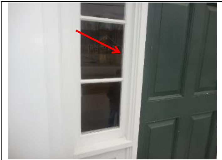
3. ACBM window glaze present on the side lights by the front entrance.
