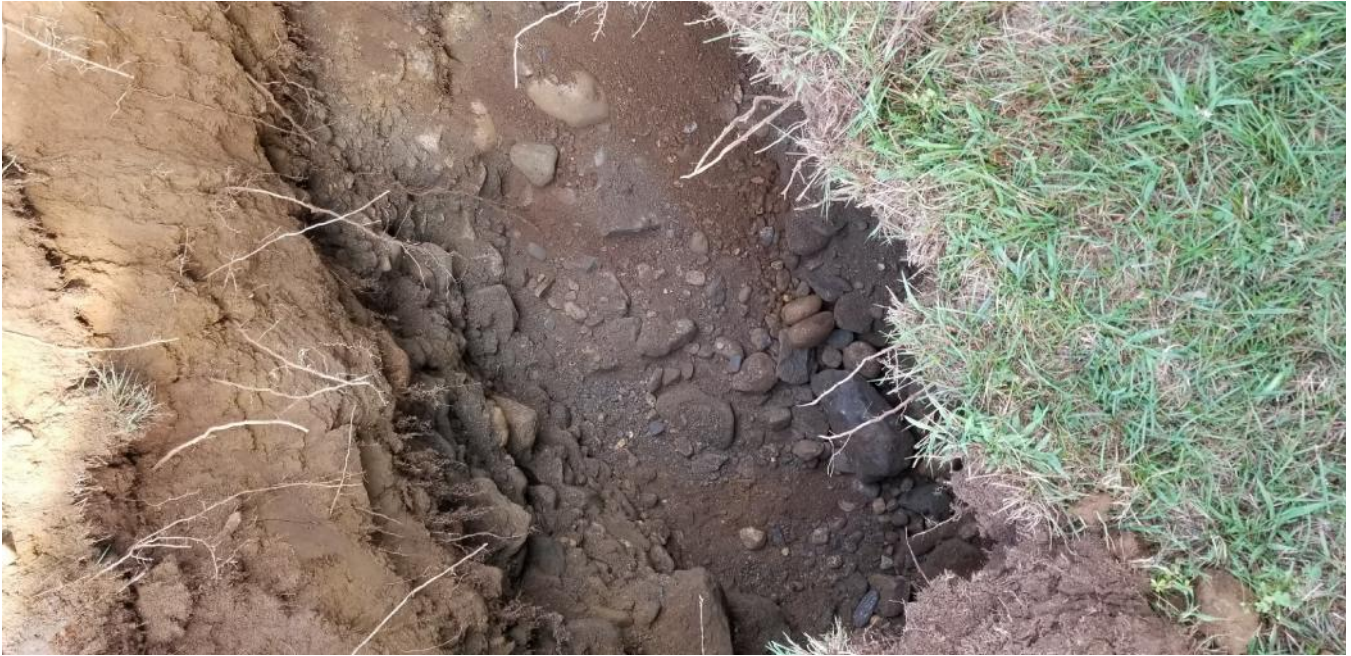
Excavation at TP-2
