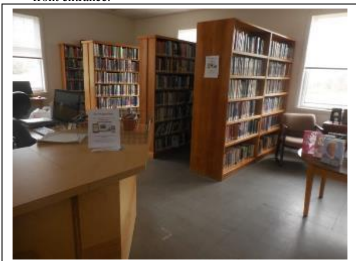
5. ACBM floor tile present throughout the 2 nd floor of the library.
