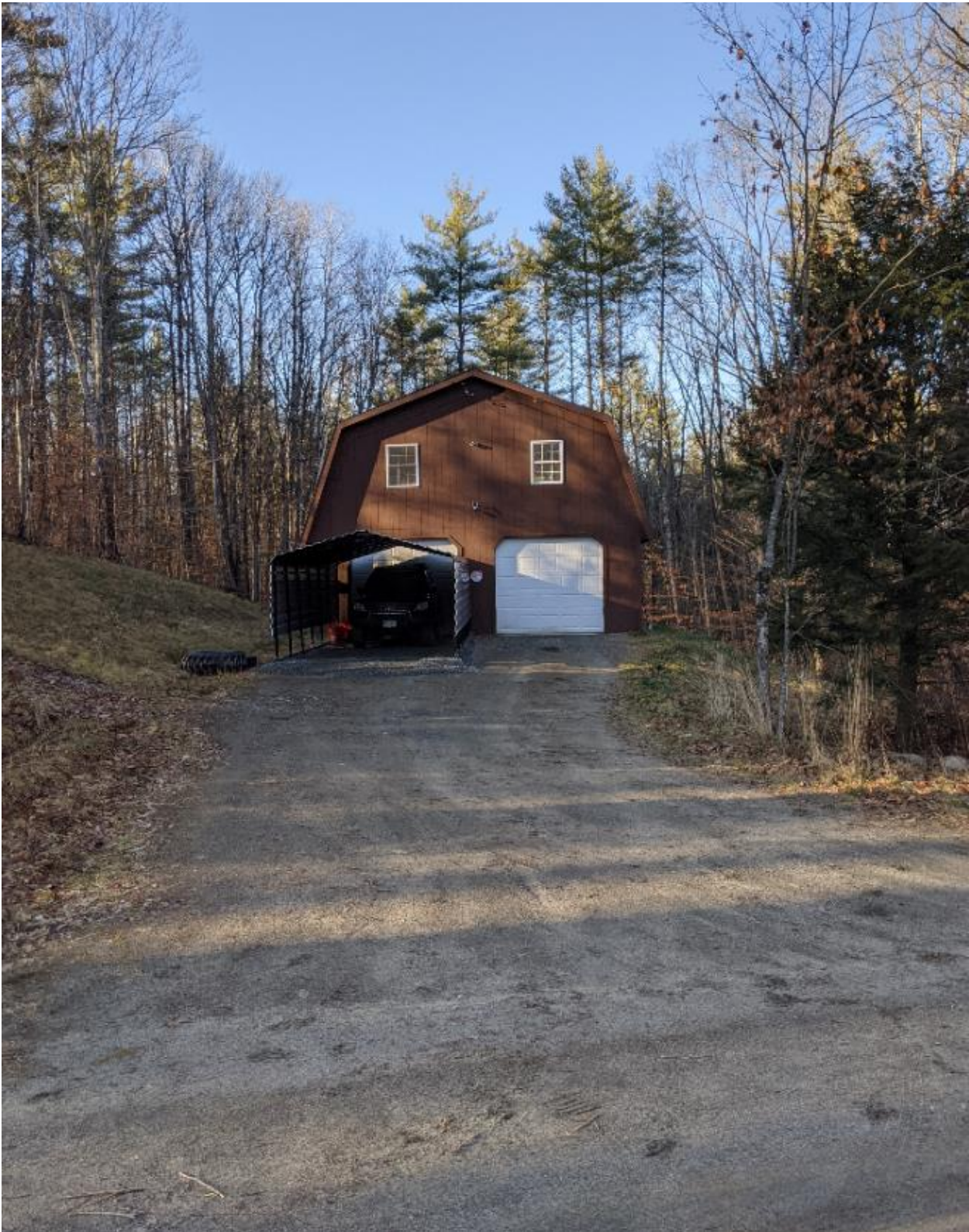
Photo of the barn from Eaton Road
