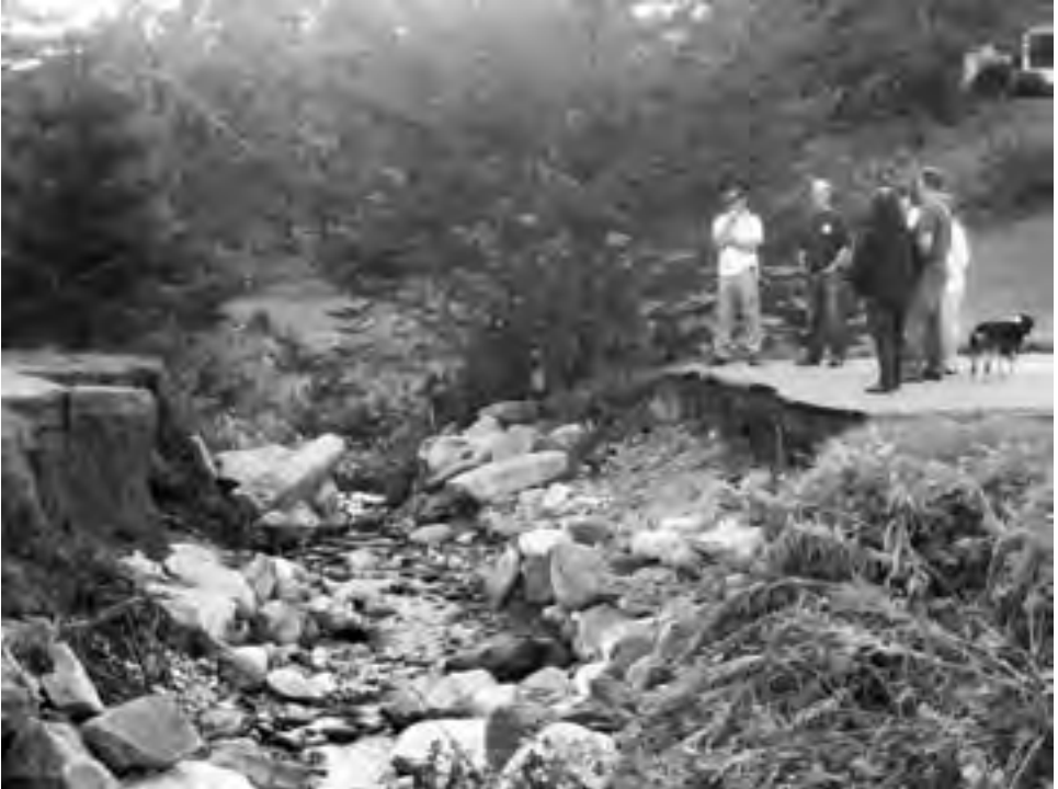
Selectboard surveys damage to Barker Road from tropical storm Irene Photo S. Halleran
