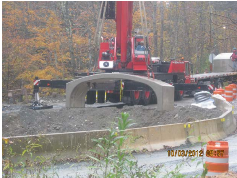
Cole Brook Box Culvert being lowered into place
