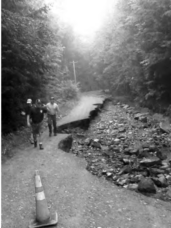
Selectman Rob Taylor, Road Agent Richard Collins and Local Contractor Scott MacLeay survey the damage to Hell Hollow Road after the July 2 nd rain storm. Photo S. Halleran
