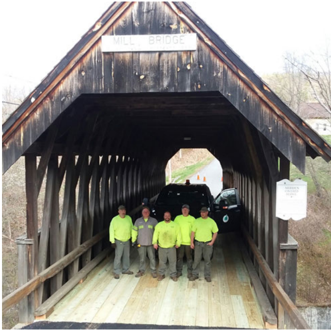
Meriden Covered Bridge 2020 (steel cleaned painted, new deck installed) Modern Protective Coatings Inc/Plainfield Highway Department
