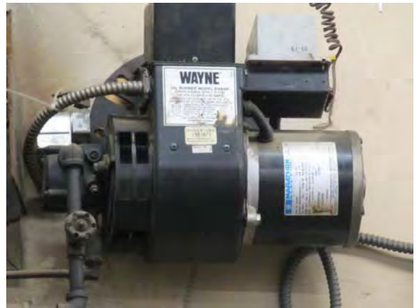
Wayne Oil Burner Model EHASR Firing Range GPS 0.75-3.00 120 Volts-60HZ-5.5 AMPS Specification Number 140-472 Serial No 1199
