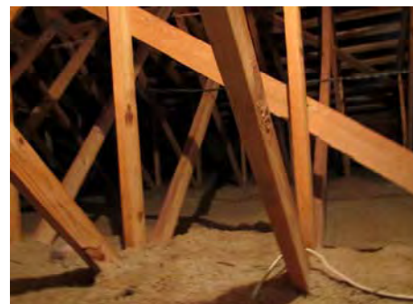
Cellulose ‘topping’ over fiberglass batts, trusses and roof strapping
